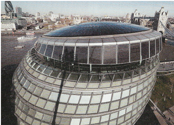
Abb.12: Solarmodule am London City Hall Building
